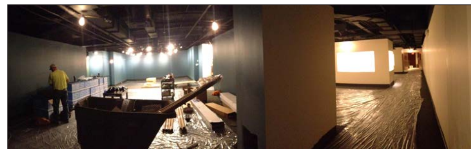
Fig. 3. Second floor galleries in Mizzou North under construction. Photo: Alex Barker.
