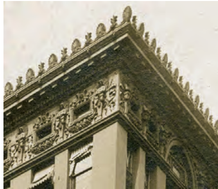
Fig. 4. The Title Guaranty Building, detail of the cornice. http://www.builtstlouis.net/opos/downtown.html .
